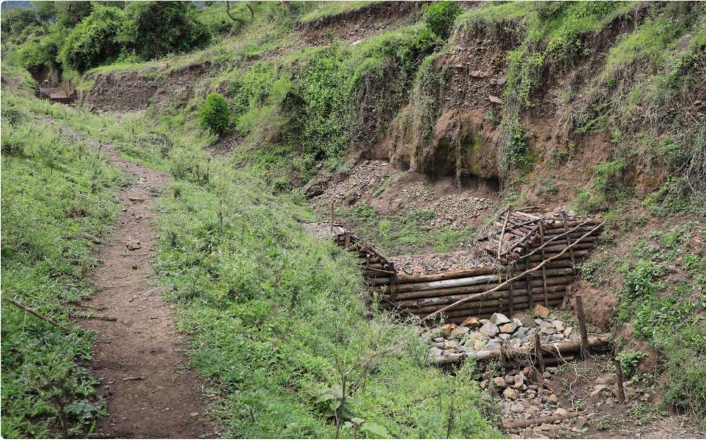
**Figure 3:** Check dam along a gully. Picture by EECMY DASSC.
