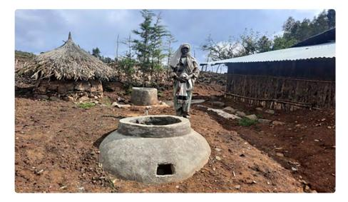
**Figure 13:** Mekoya Kassaw and her biogas digester. In addition to cooking, biogas leftover is used in their farm to improve the fertility of the soil and hence crop yield. Picture by Wandem Feleke EECMY DASSC.
