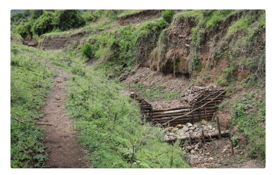
*Figure 3:* Check dam along a gulley. Picture by EECMY DASSC.
